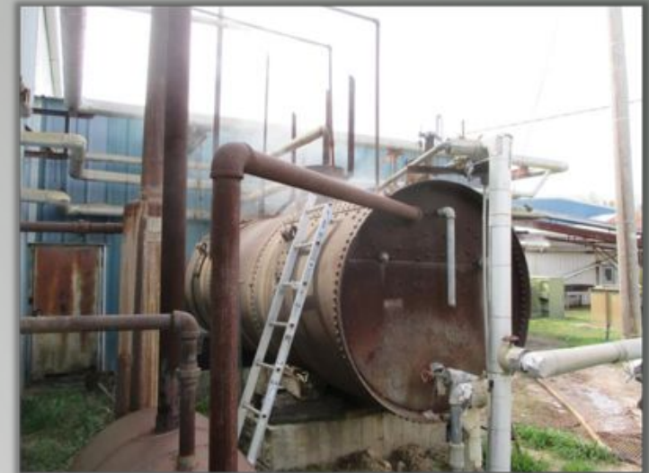
Uninsulated condensate tank, with openings in the top
